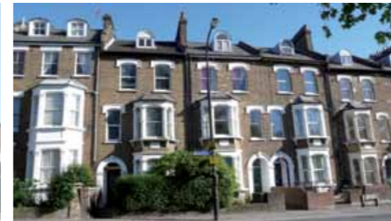
07 4 Storey Victorian terraces further along Iverson Road
